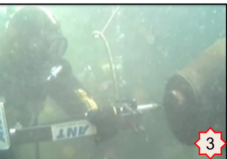
Positioning of the MULTIFLEX Circular Cutter
